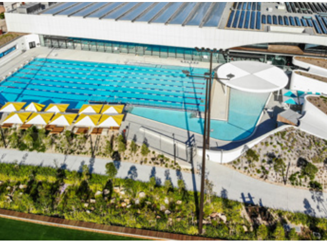
Gunyama Park Aquatic Centre Photo: Chris Southwood / City of Sydney
