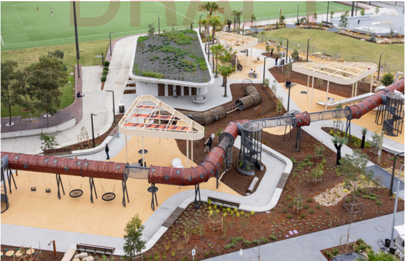
Gunyama Park stage 2 Photo: Chris Southwood / City of Sydney
